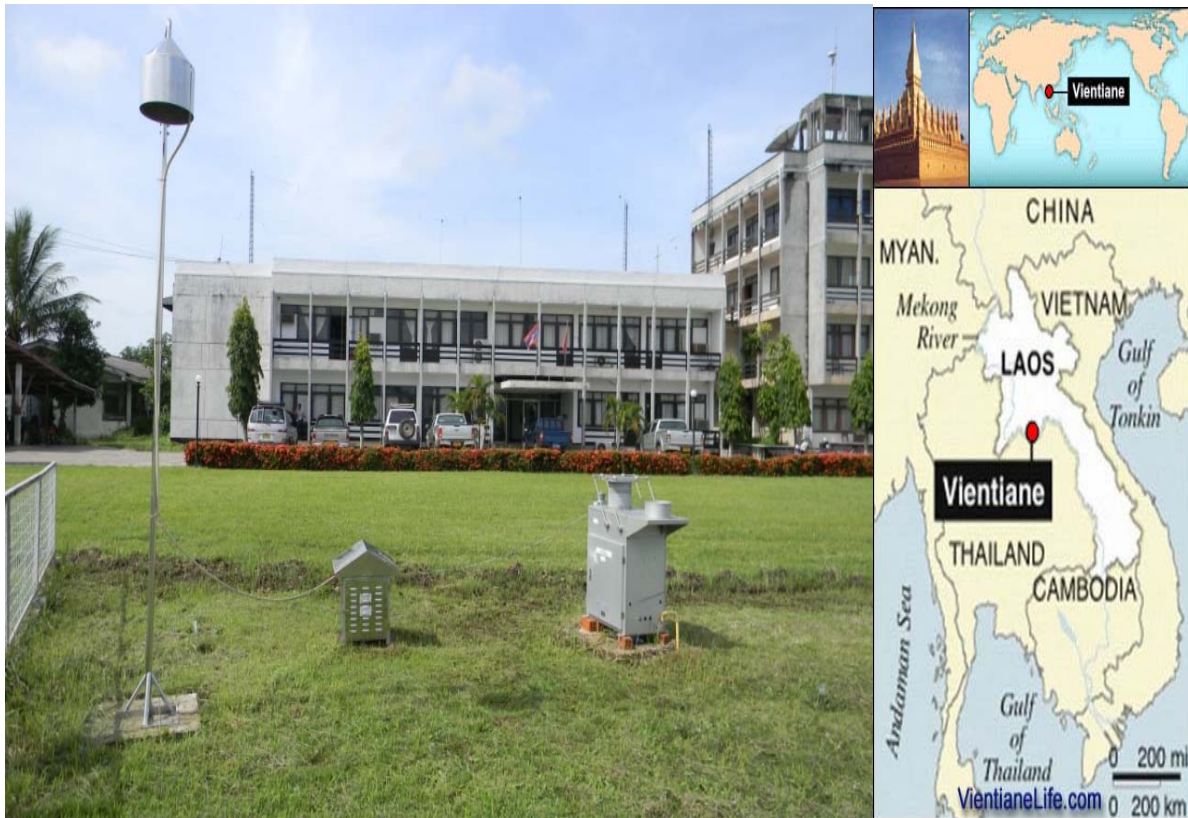
Figure 1.1.1. Monitoring station for wet and dry deposition.
