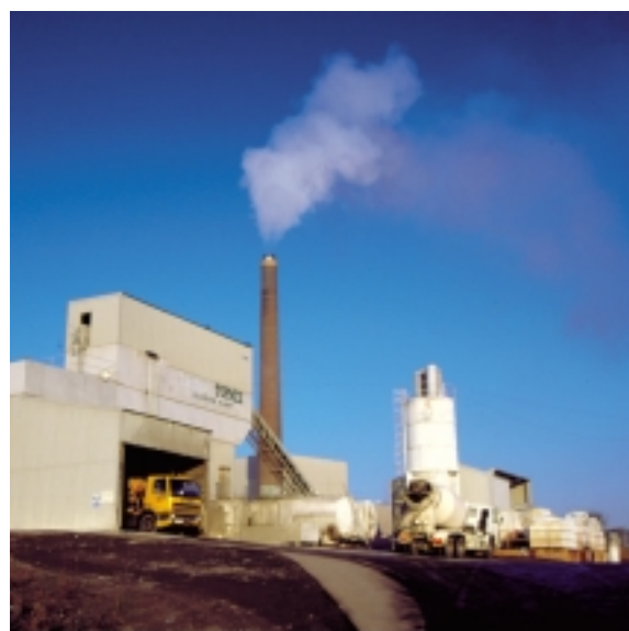
Cement Batching Plant, Part B Process
