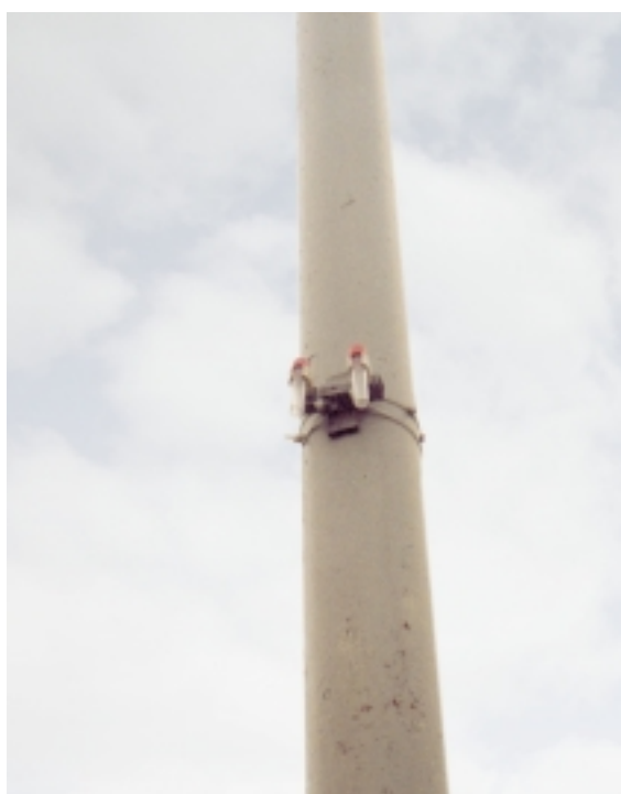
Passive Monitoring Using Diffusion Tubes
