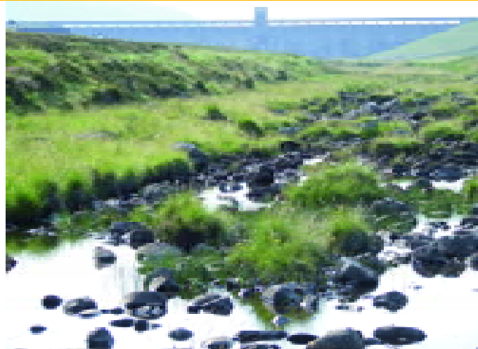
Glascarnoch River below the hydropower dam, showing changes to the river channel due to lack of compensation flows from the reservoir
