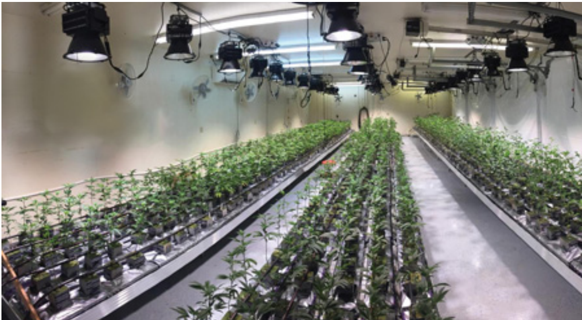
FIG. 2. Spectrum King LED luminaires use predominantly white LEDs and are regularly sold into legalized medicinal or recreational cannabis growing operations indoors.
