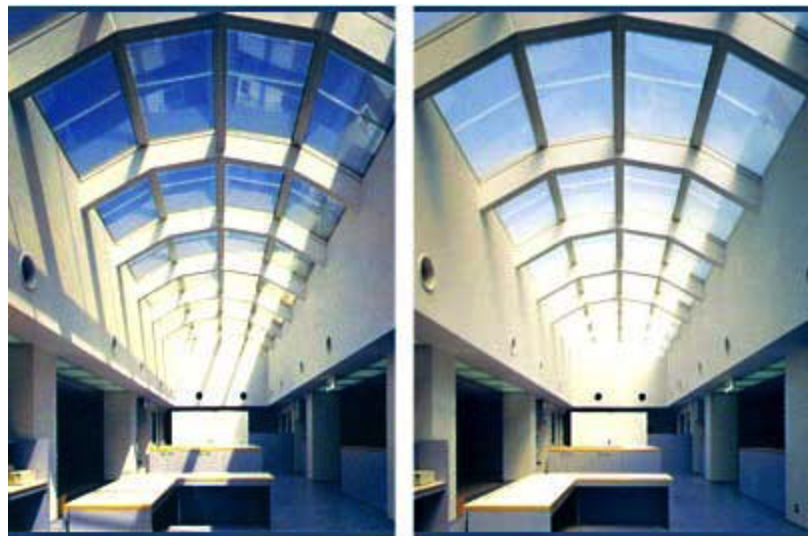
These roof panels are fitted with SwitchLite Privacy Glass™. PHOTO COURTESY SWITCHLITE PRIVACY GLASS™
